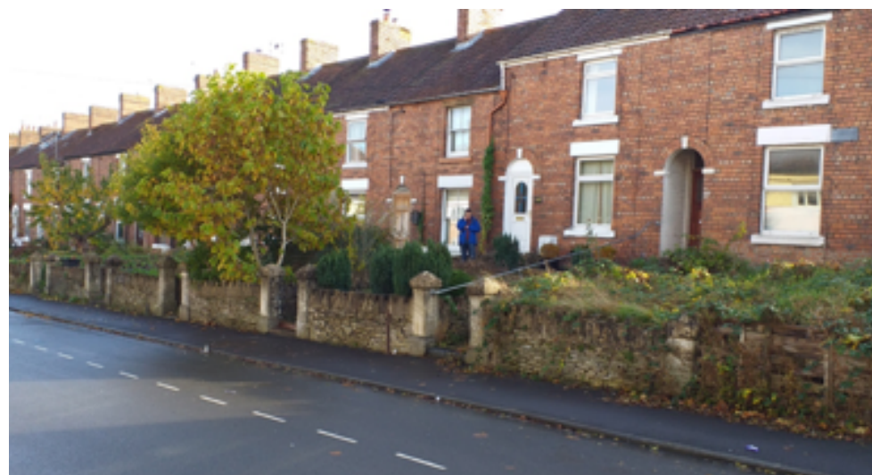
Below: Decorative English Bond brickwork of the early 20th Century Blackmore Terraces on Forest Road
