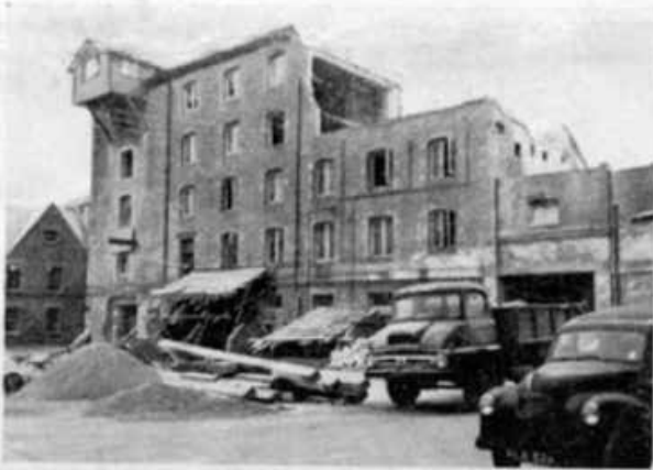
1961. The top three storeys come off. . . . .
