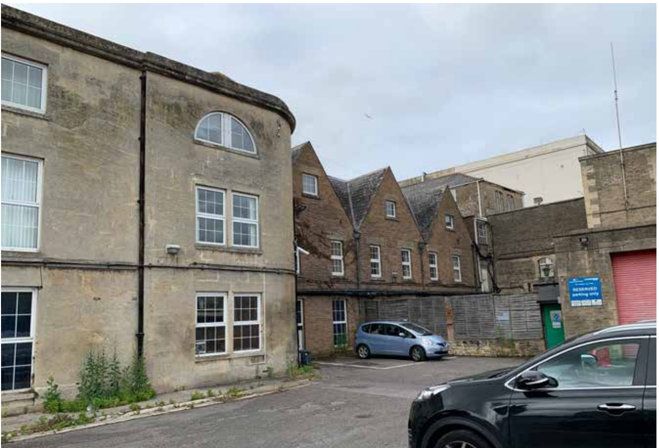
3.3 Avon House and 17 th century gabled range to rear
