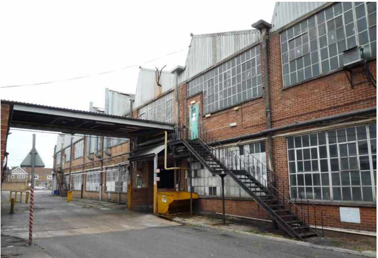
3.23 Main Production Hall
