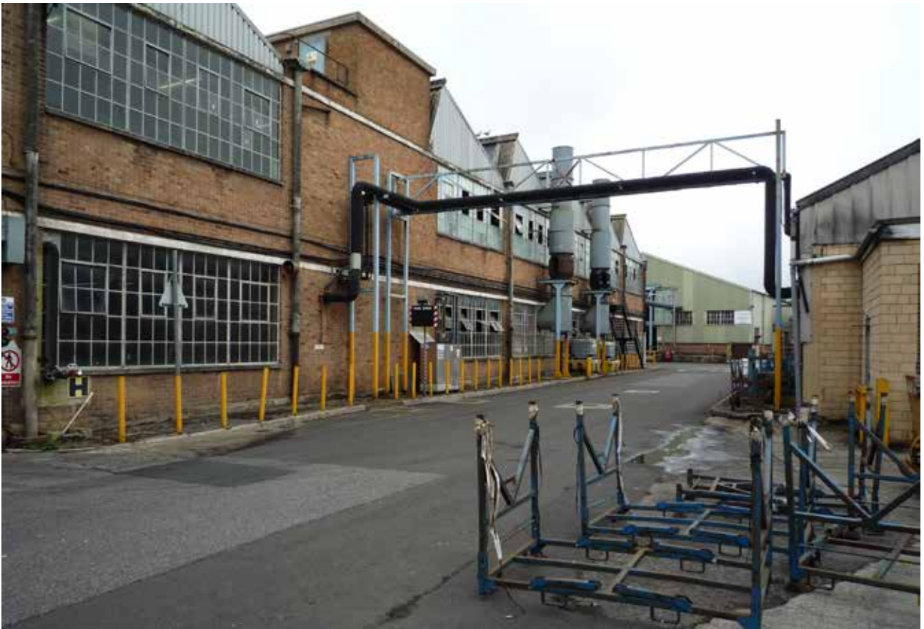
3.24 Main Production Hall
