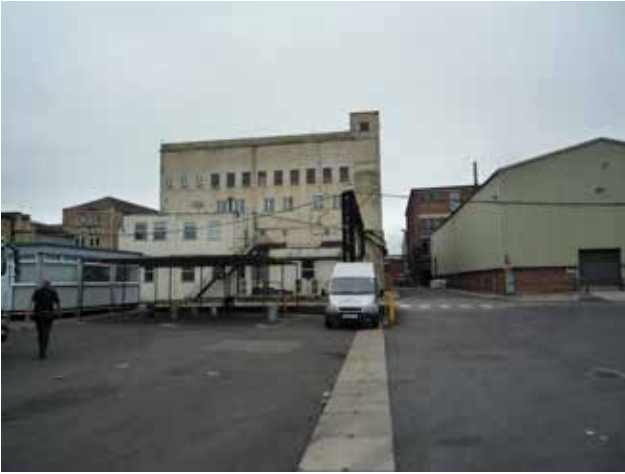
3.11 1920s Office Building
