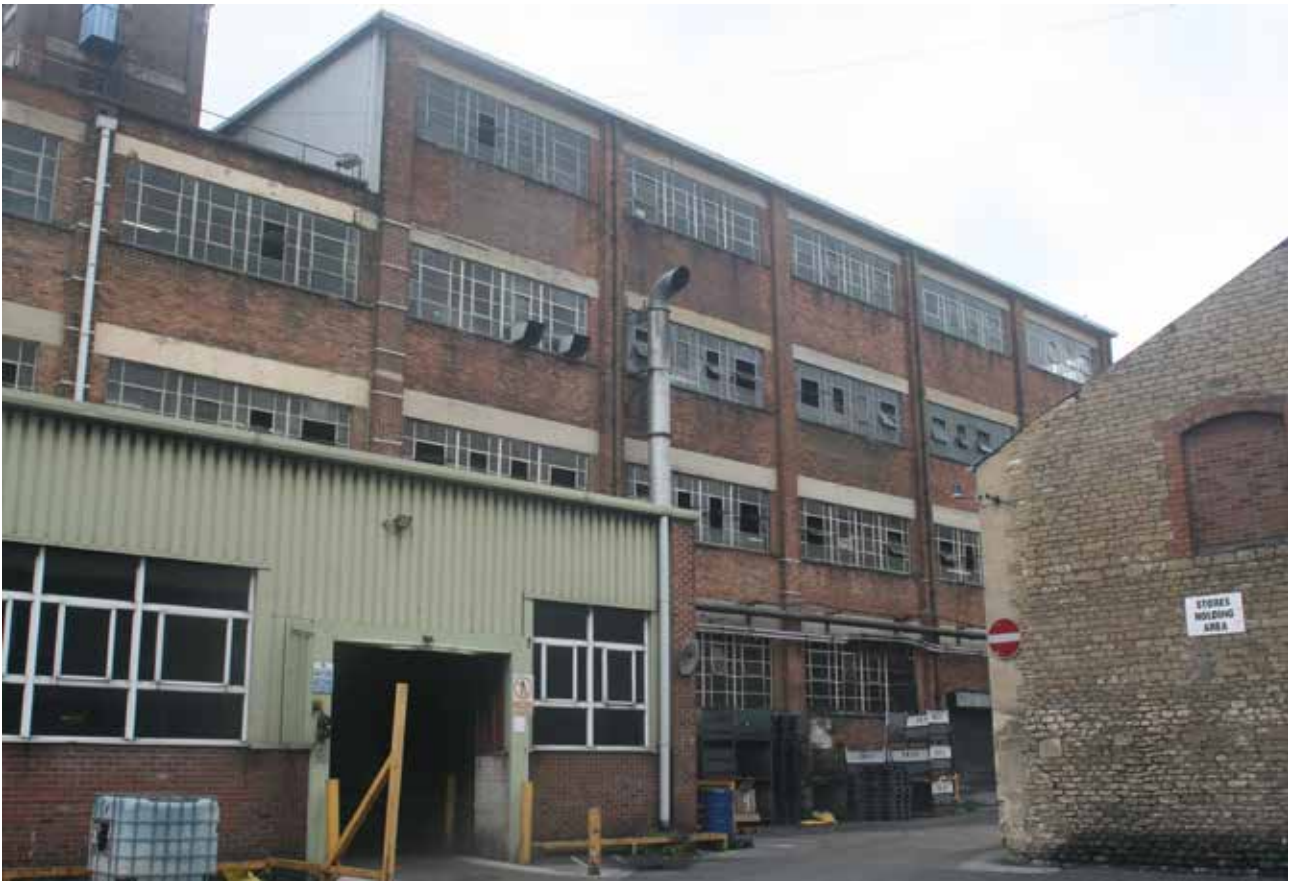
3.20 Main Production Hall
