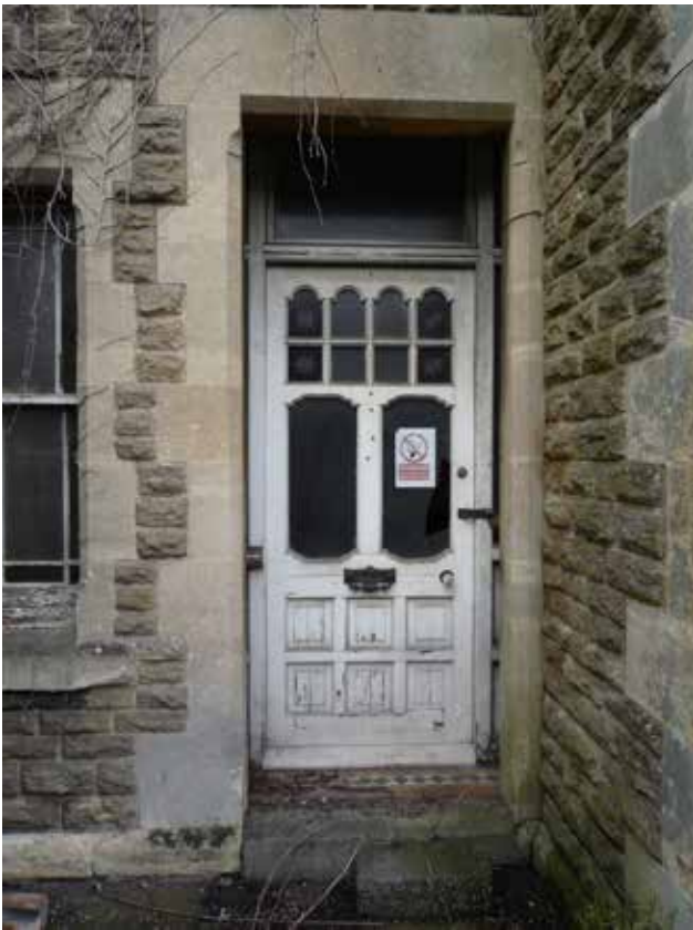
3.19a Front door detail 13 Beanacre Road
