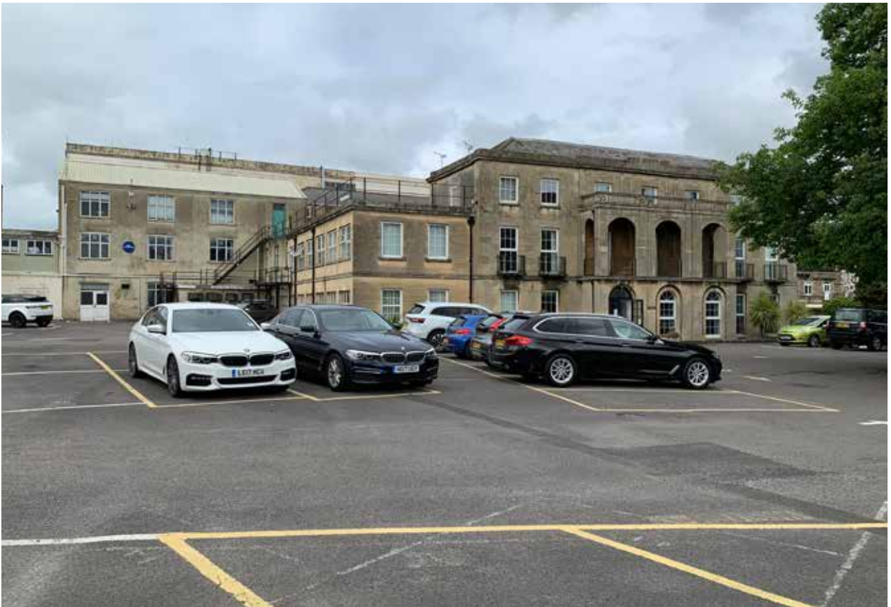
3.2 Avon House and mid-20 th century extension to west
