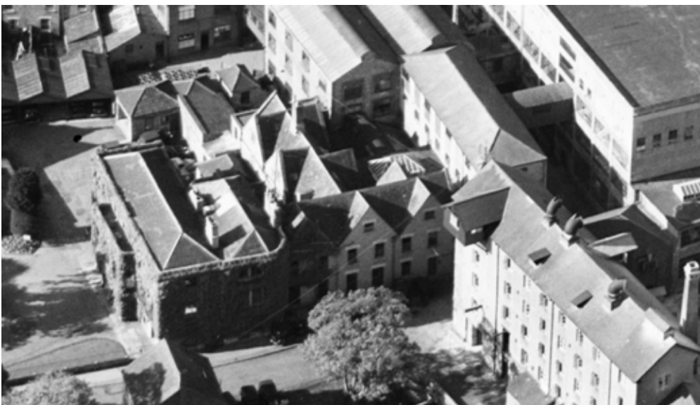
2.19 1950 aerial photograph of Avon House from the east, before 1950s alterations. (Historic England EAW 033282)
