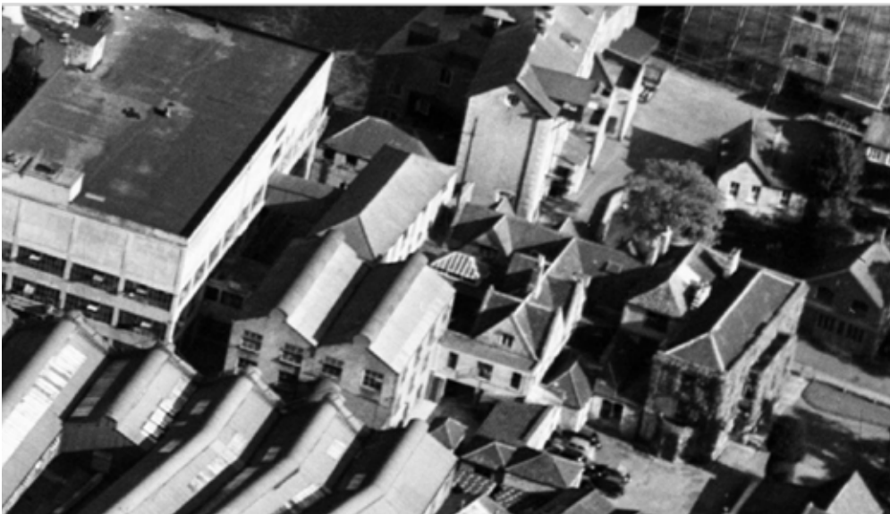
2.18 1950 aerial photograph of Avon House from the west, before 1950s alterations. (Historic England EAW 033279)
