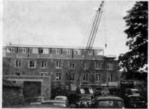
. . . . . and in 1964 another storey goes on.
