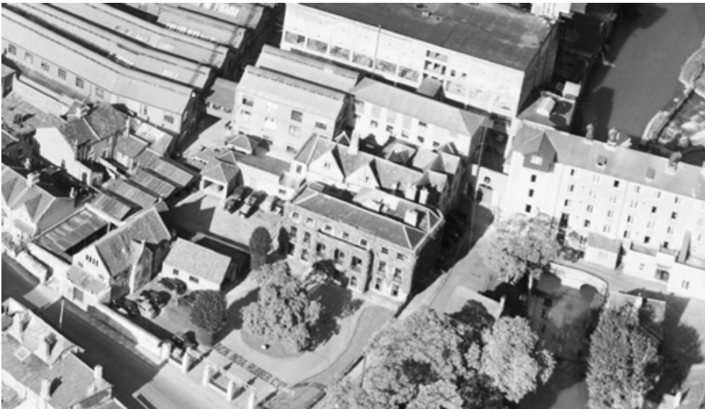
2.17 1950 aerial photograph of Avon House from the south east, before 1950s alterations. (Historic England EAW 033273)
