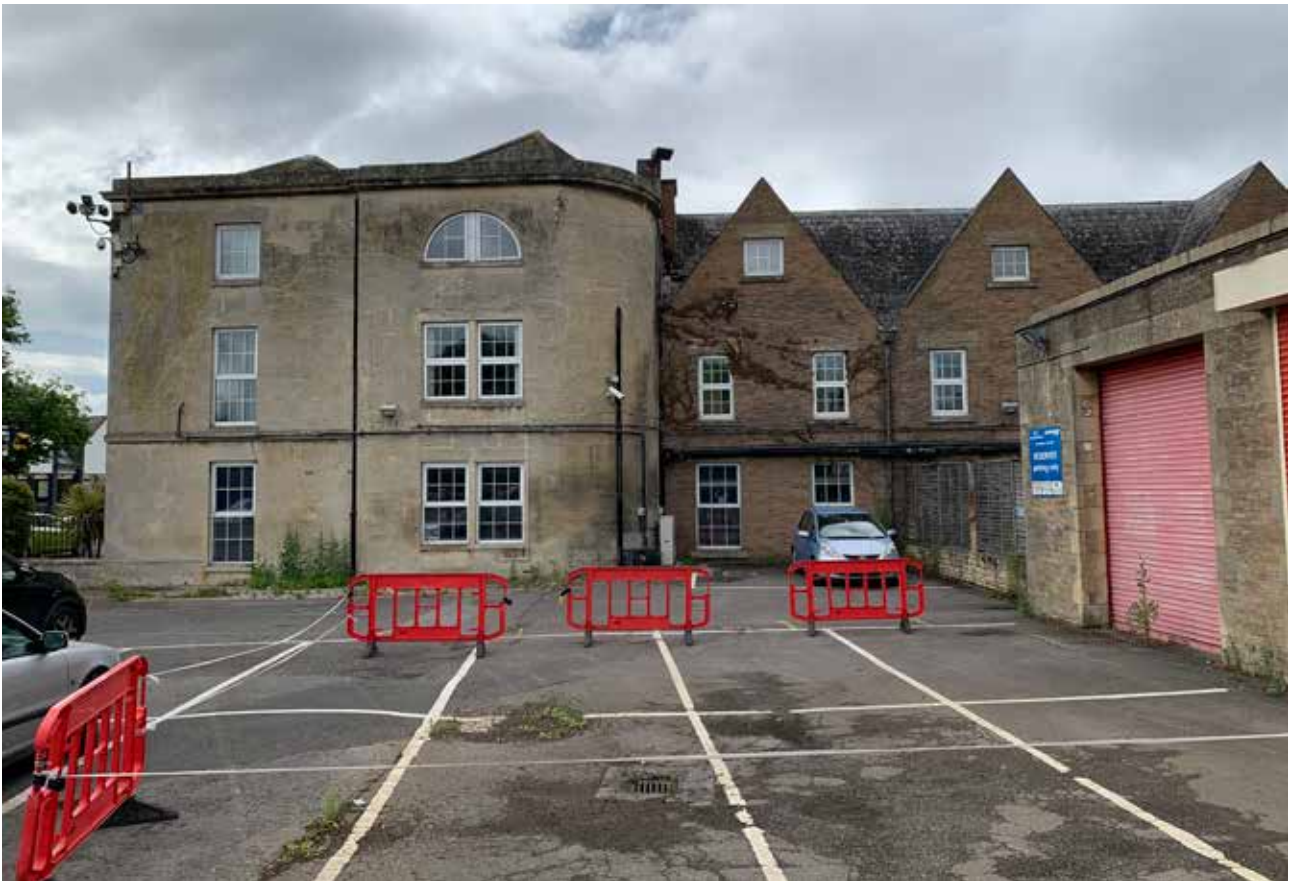
3.4 Avon House and 17 th century gabled range to rear
