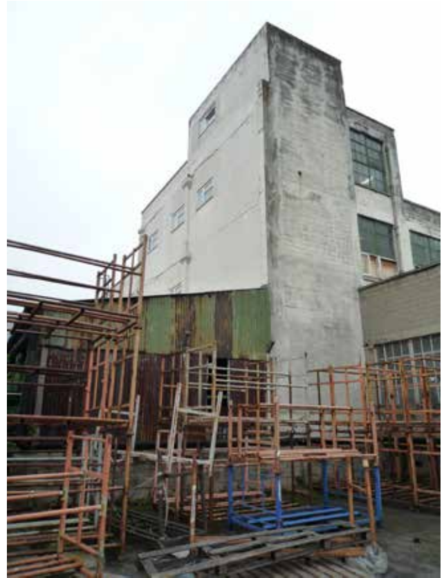
3.12 1920s Office Building
