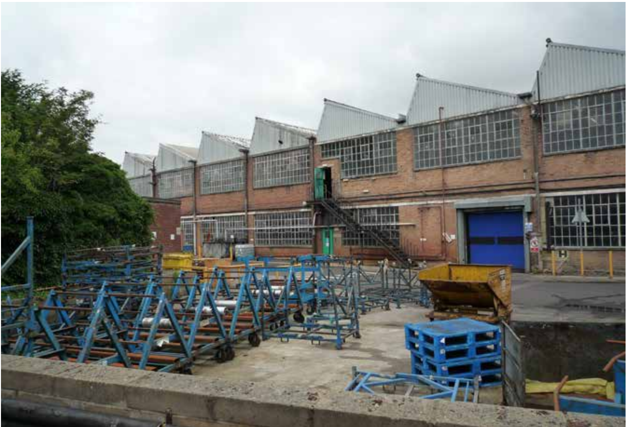
3.22 Main Production Hall
