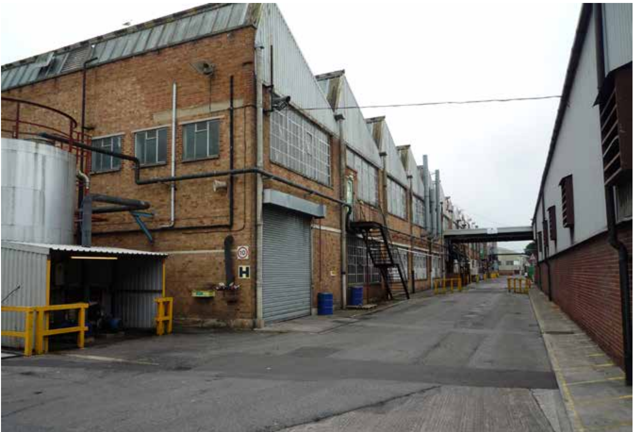
3.25 Main Production Hall
