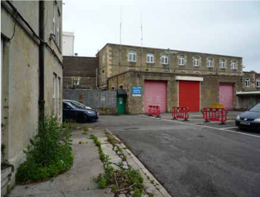
3.17 Former Fire Station
