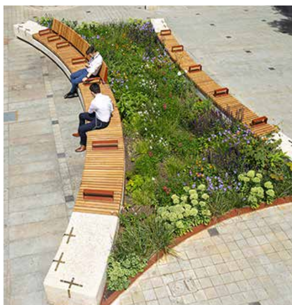
Figure 46: Raised planter with integrated seating
