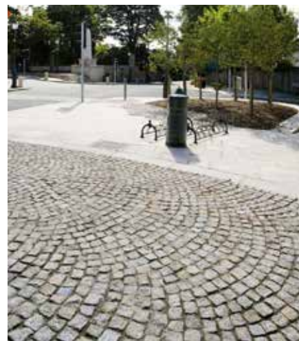
Figure 39: Clear paving transition, and use of traditional cobblestones to slow down traffic
