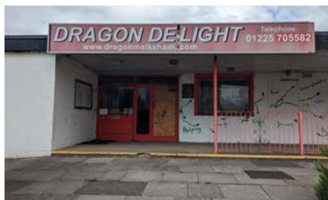
Figure 12: Former chinese take away site
