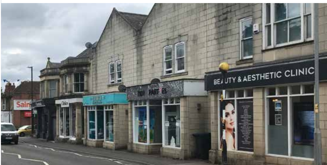
Figure 25: Consistent, but tired shopfronts, Bath Rd
