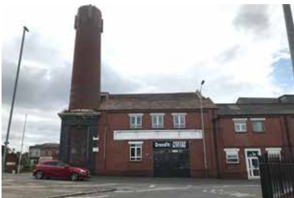
Figure 105: Typical Victorian red brick with clay pantile roof
