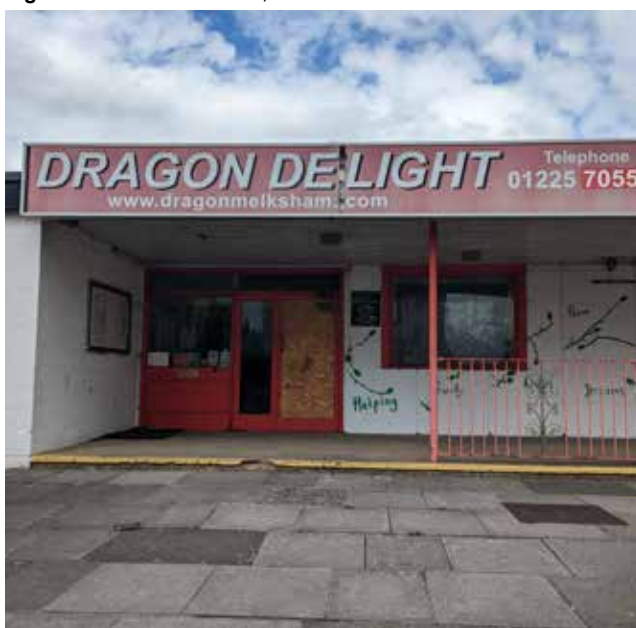
Figure 93: Vacant take away / restaurant unit
