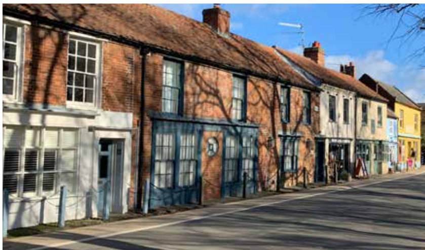
Figure 38: Unified, vibrant signage, in keeping with local character, Burnham Market
