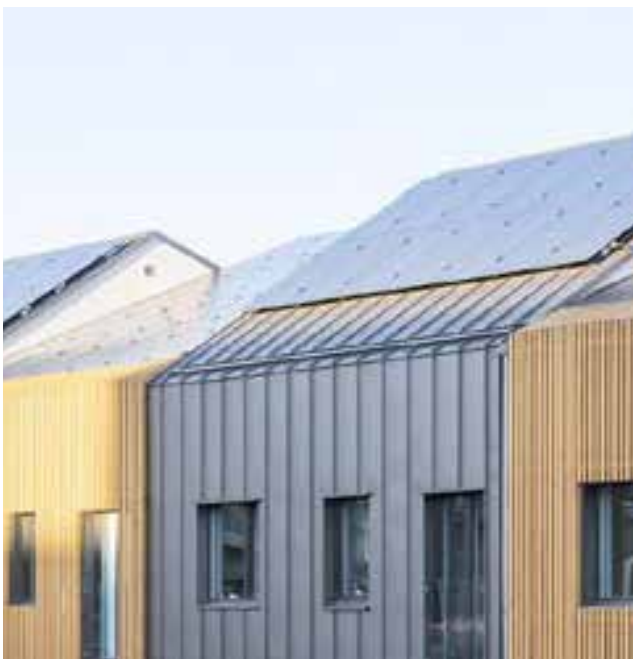
Figure 52: PV cells on pitched roof
