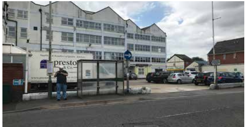
Figure 106: Typical gabled roofline
