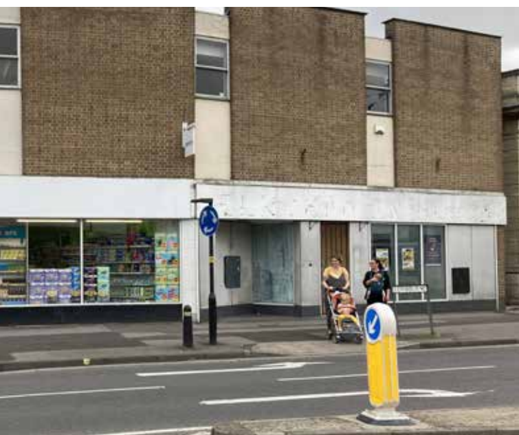
Figure 96: Former Nat West bank, Lowbourn
