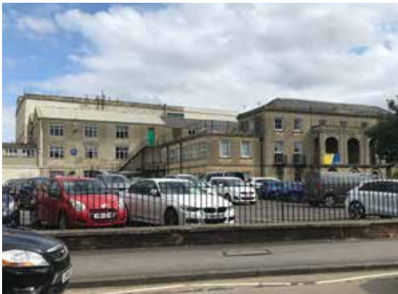
Figure 104: Grade II listed Avon House
