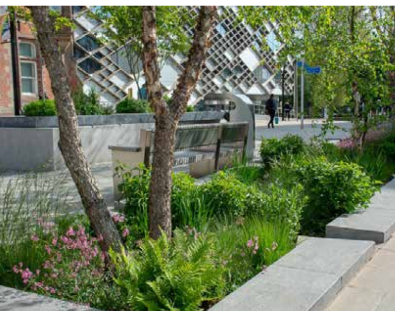
Figure 47: Raingardens with outlet kerb in stone
