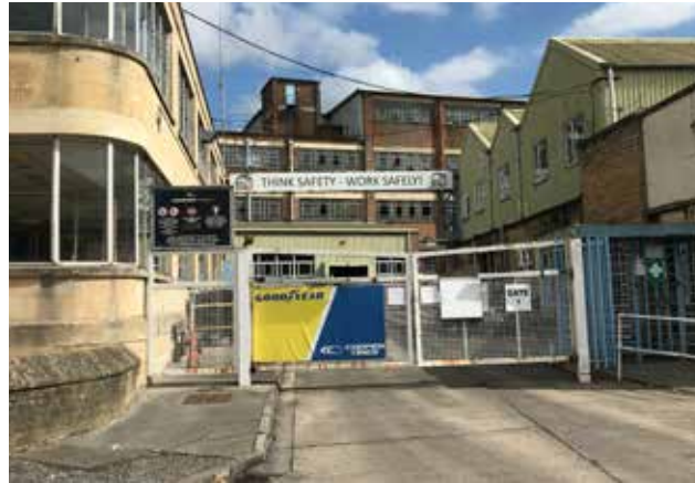
Figure 72: View of a variety of industrial building styles, including stone, red brick and green corrugated steel cladding.
