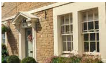
Figure 30: Light coloured rendered window frame and sash window with vertical panelling.
