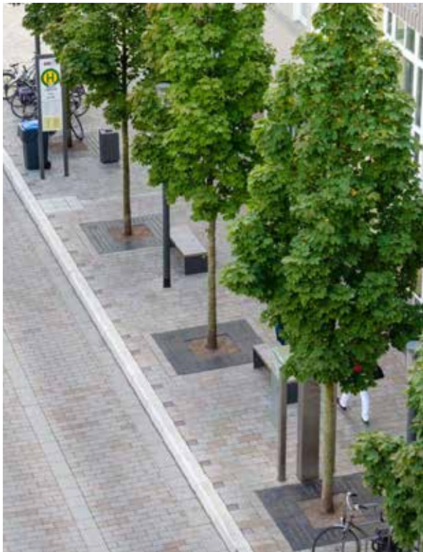
Figure 137: Example of street trees in contained tree pits
