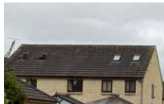
Figure 57: Rooflight on gabled slate roof
