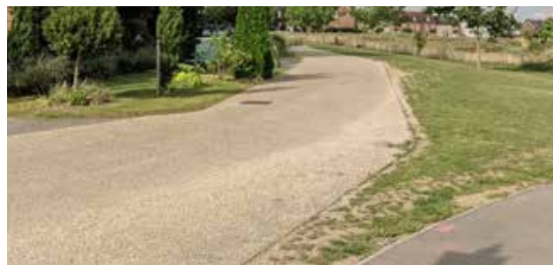
Figure 102: Above, positive examples of permeable paving. The top and middle photo show examples of paving that could be used within the built environment, whilst the photo to the bottom shows an example of edge lane that uses gravel, in earthy palette, which could also be used in footpaths within the countryside.
