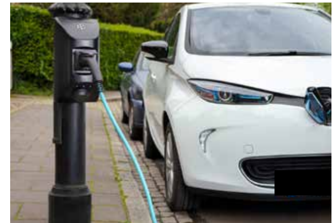
Figure 116: Example of on-street electric vehicle charging points.
