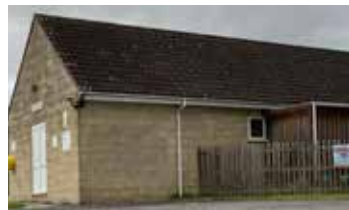
Figure 49: One storey, stone render building with pitched roof.
