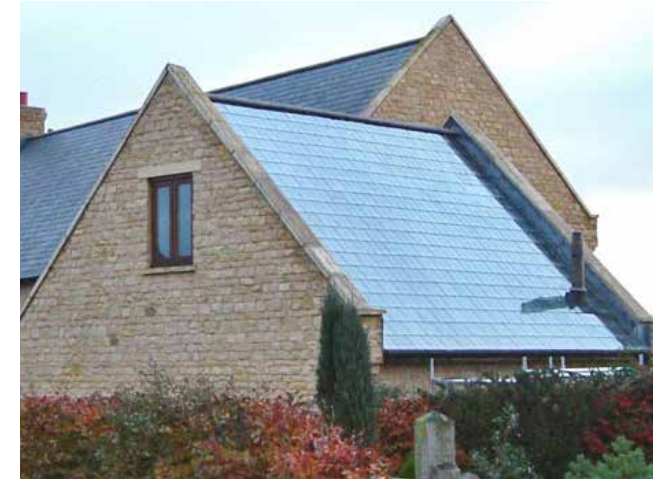
Figure 154: Positive example of implementing solar panels since the design stage, elsewhere in the UK.
