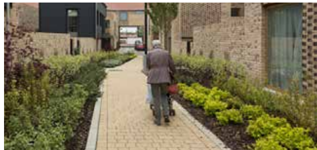
Figure 103: Example of footpath that uses impermeable paving which should be avoided.
