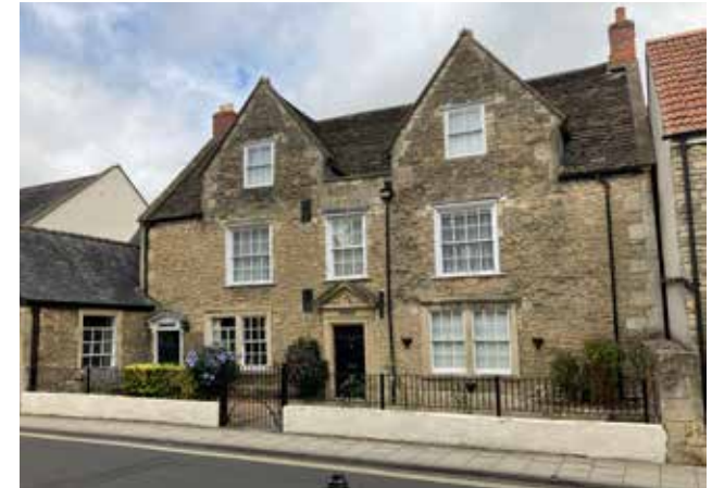
Figure 182: A positive local example of a house with dark clay tiled gabled roof and dormer windows, buffered by a mixture of vegetation, low wall and iron fencing, sash windows and stone construction with ashlar stone quoin detailing.
