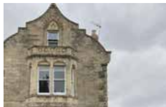
Figure 41: Ashlar stone, Dutch gable roof and 2 storey canted bay windows.
