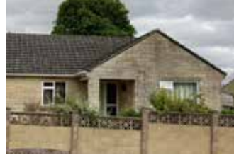
Figure 52: Dark clay pantile cross-gabled roof.
