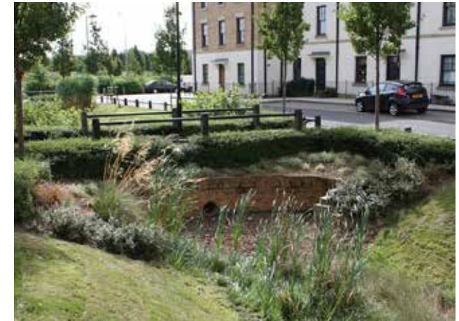
Figure 144: Example of swales check dam integrated with a crossing point, elsewhere in UK.
