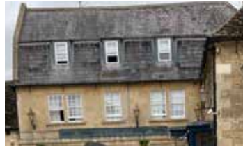
Figure 33: Ashlar stone with mansard roof in Welsh slate.
