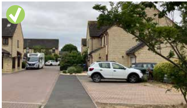
Figure 117: Local example of a small parking court in a cul-de-sac in Melksham which uses permeable material.
