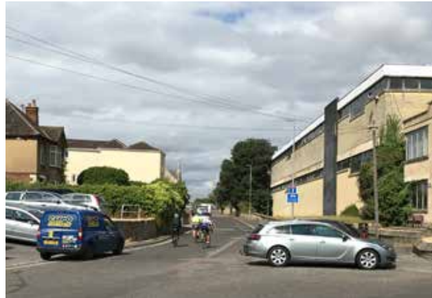
Figure 68: Four storey industrial building facing onto The City and Bath Road
