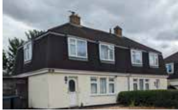
Figure 50: Mansard roof with dark clay tiles and rendered facade.
