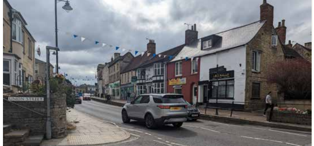
Figure 06: View of Bank Street.
