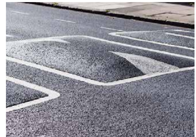
Figure 107: Example of a speed cushion.
