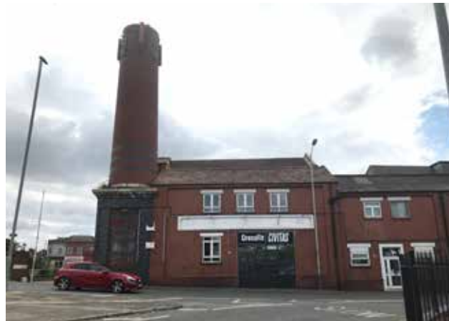
Figure 74: Red brick with clay pantile roof and red brick tower.
