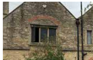
Figure 40: Light-leaded window with red brick detailing above.
