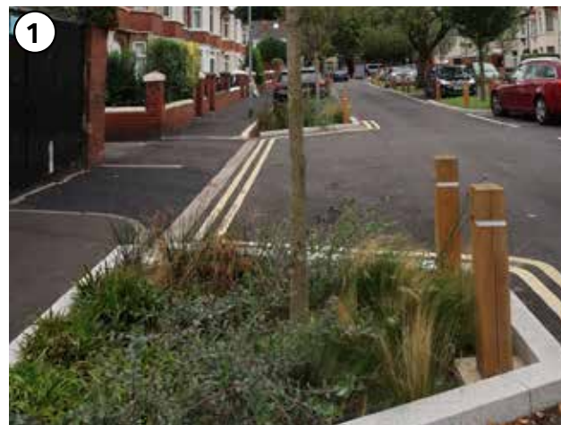
Figure 128: Example of a bioretention tree along a residential street. Those trees could also be retrofitted into existing roads.
