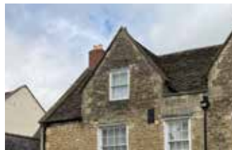
Figure 28: Attic dormers with white framed sash windows.
