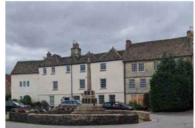
Figure 183: Positive local example of a clay tiled gabled roof terraced house with stone and off-white render, vertical sash windows and chimney stacks which interrupt the roofline.
