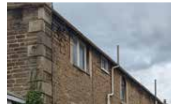
Figure 39: Ashlar stone quoins.
