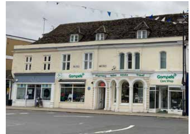
Figure 193: A local example of a well-laid out shopfront, white front painted timber finished window and door frames and clear signage positioned on fascia, Bank Street
