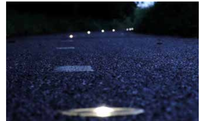
Figure 202: Example of a foot/cycle path which is lit by solar cat's-eye providing some light for pedestrian and cyclists without creating any disturbance to the nearby properties or unacceptable levels of light pollution.
