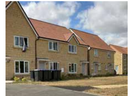
Figure 67: Gault brick with red clay pantile roof and repeated architectural style
