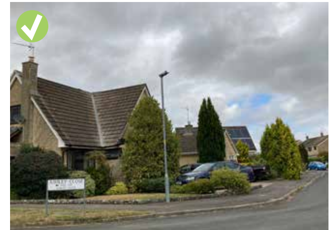
Figure 113: Local example of on-plot front parking with vegetation to provide screening. This parking solution avoids cluttering the front façade of the house.
