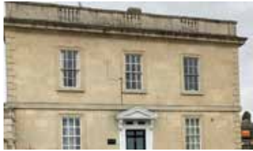
Figure 27: Ashlar stone with rusticated quoins and moulded cornice and parapet with flat roof.
