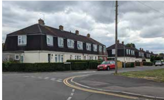
Figure 42: Linear form and consistent building line with small set back from the road in the town centre, Milton Avenue.
