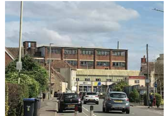
Figure 71: Flat roofline of an industrial building.
