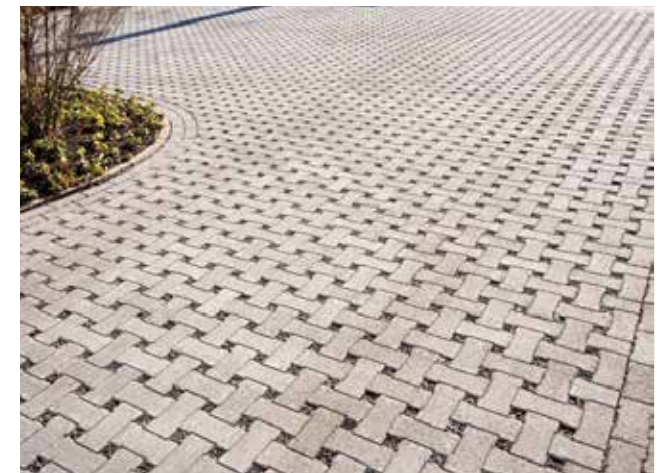
Figure 150: Example of a permeable paving that could be used from driveways.
