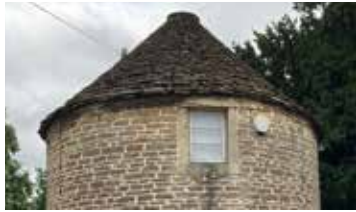
Figure 32: Coursed rubblestone with slate tiled conical roof.
