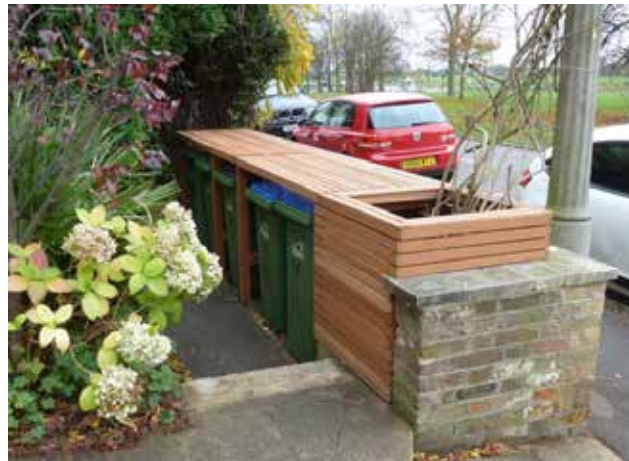
Figure 121: Example of wheelie bin storage for front gardens that include a green element to improve the aesthetics.
