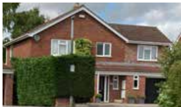
Figure 48: Red brick with cross-gabled, clay pantile roof and hedgerow boundary treatment.
