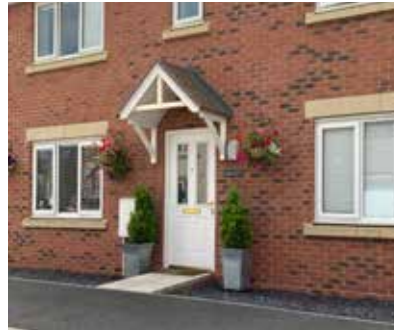
Figure 62: Red brick with gabled roof over the door and white casement windows.
