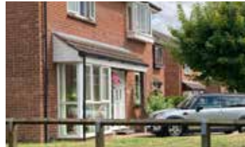
Figure 47: Red brick and porch with glazing and sloped, dark clay pantiled roof.
