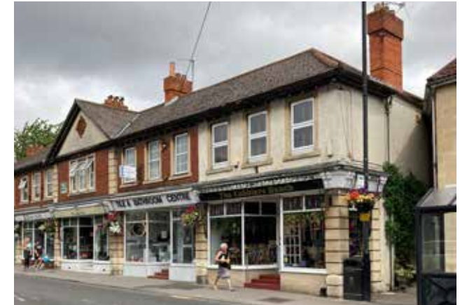
Figure 192: A local example of a well-laid out shopfront, with white painted timber finished window and door frames, and clear signage positioned on fascia, Bath Road.
