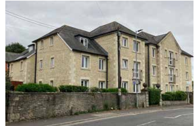
Figure 168: Local example of a higher density 3-storey apartment block in Melksham town centre.
